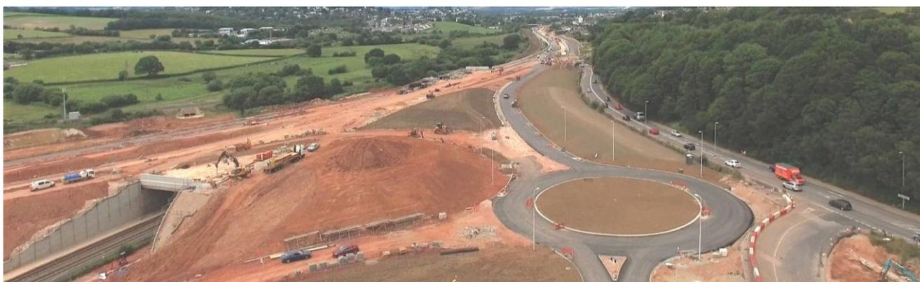
At the southern end of the project we have begun preparatory works for the new traffic light-controlled junction near Kerswell Gardens at the bottom of Hamelin Way. This phase of works will take approximately 14 weeks to complete. A series of traffic realignments will be taking place during the works in order to maintain access to all routes.
