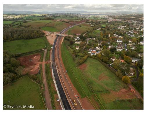
construction team can turn their attention to peripheral works. These will continue along the length of the project well into 2016. The works include the continuation of Aller Brake Road through the Romany Jones layby to join up with the existing A380. This particular phase of work is being done only after the main line opens and the current road becomes guieter.
